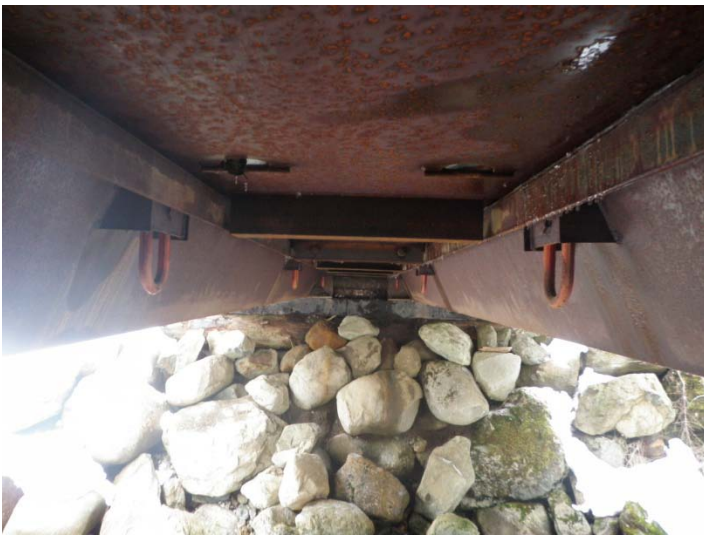
Cover plate in-between 2 box girders
