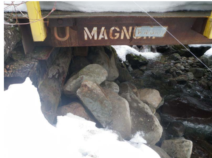
Town riprap angle
