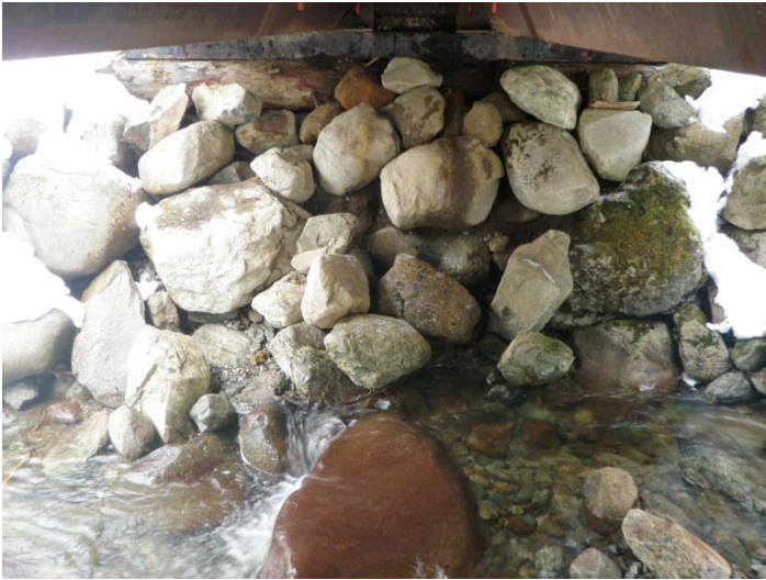
Town abutment and riprap
